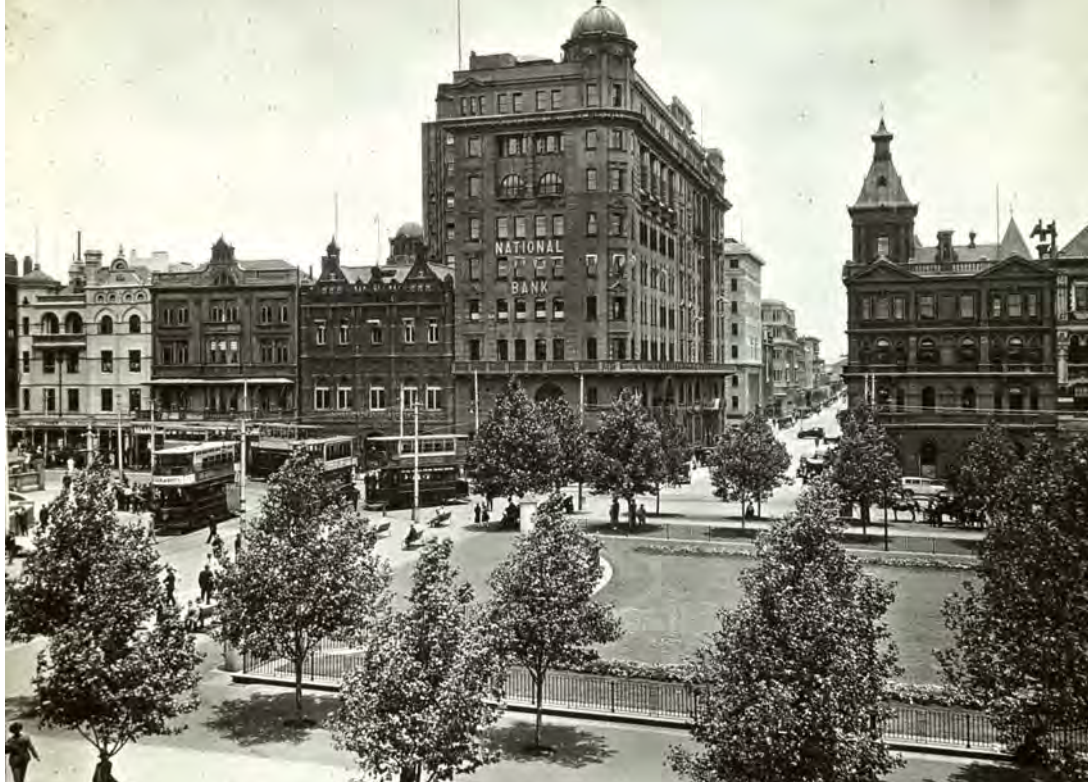
▲ Image 3: National Bank building, Cape Town c1920-c1930 (Linton Brothers, photographer). State Library of Victoria Picture Collection, Accession No: H92.339/84
